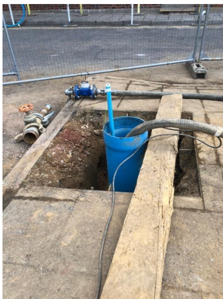
BH2 during well development
