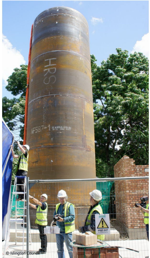
[below] Figure 16: Thermal storage completed installation at Bunhill Energy Centre
