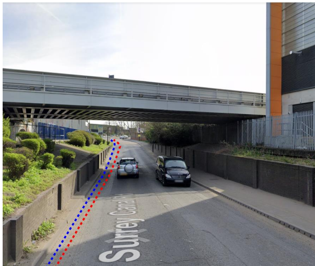
Figure 31. Surrey Canal Road and retaining wall including indicative location of proposed pipes (looking east). Image: Google Streetview
