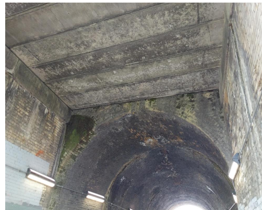
Figure 27. Arch 95 / 95A precast beam extension
