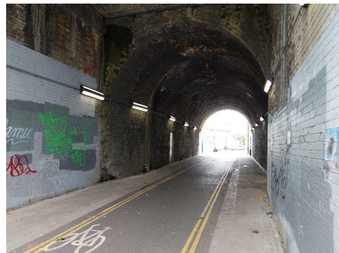
Figure 15 Area beneath the archway (5b)
