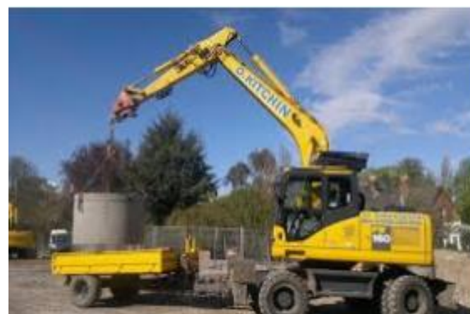
Figure 36 - "rubber duck" excavator
