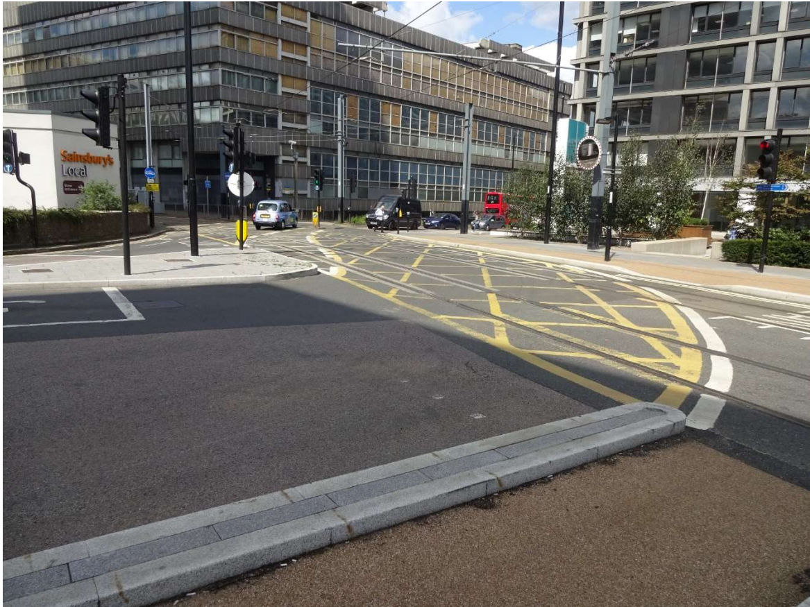
Figure 13 Looking north-west at Tram crossing where Addiscombe Grove becomes Cherry Orchard Rd
