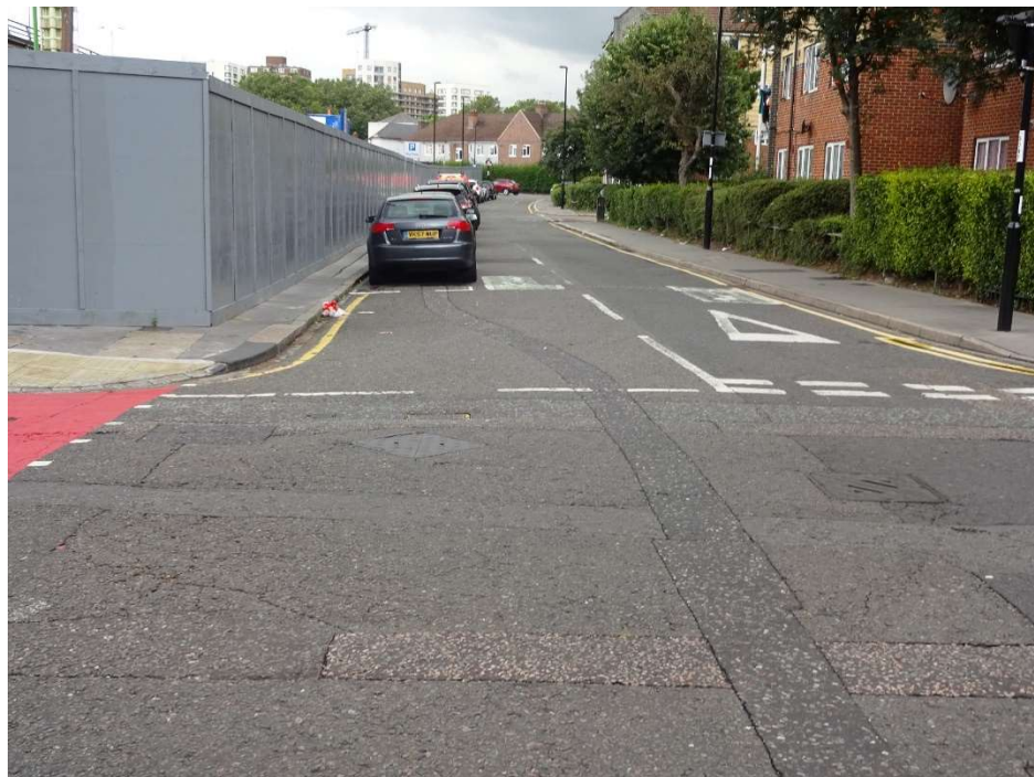
Figure 29 Scarbrook road at Wandle Intersection Looking SOUTH WEST
