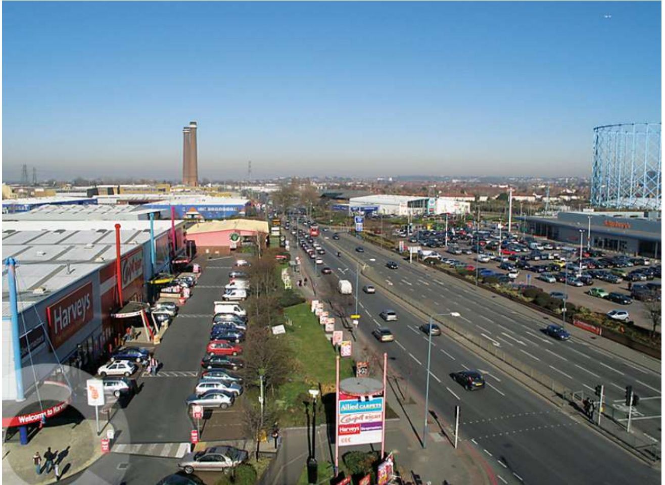
Figure 3-13 – Purley Way (A23) Looking North
