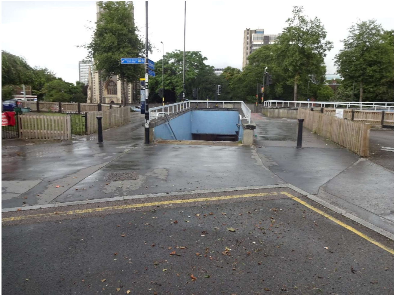
Figure 3-18 – Roman Way Underpass Entrance
