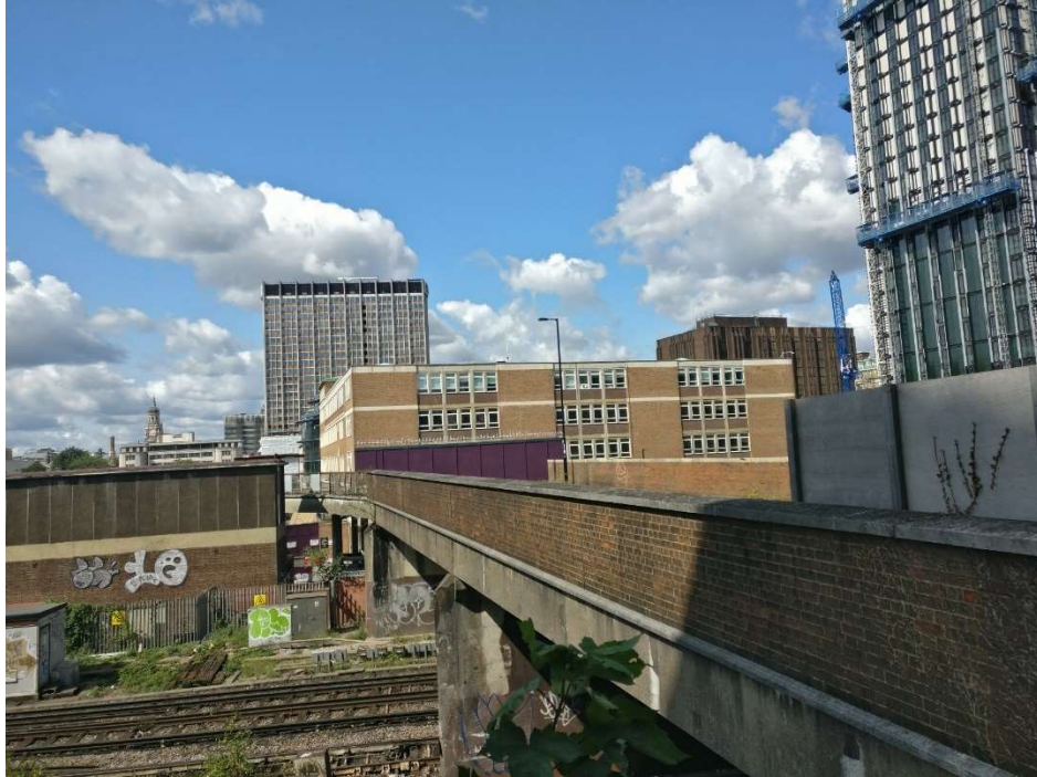
Figure 10 Looking west across the Bridge from Hazledean Rd
