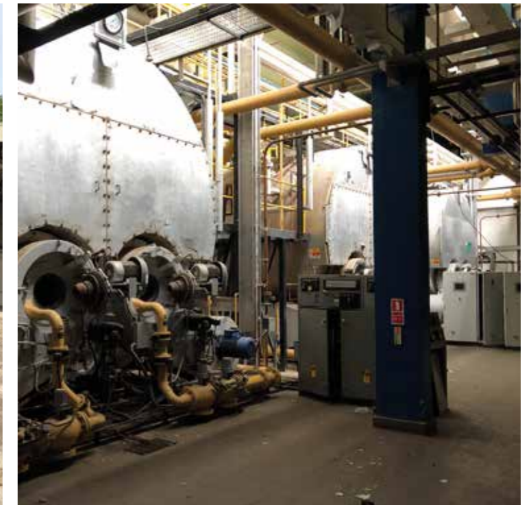
Stripout in progress at energy centre
