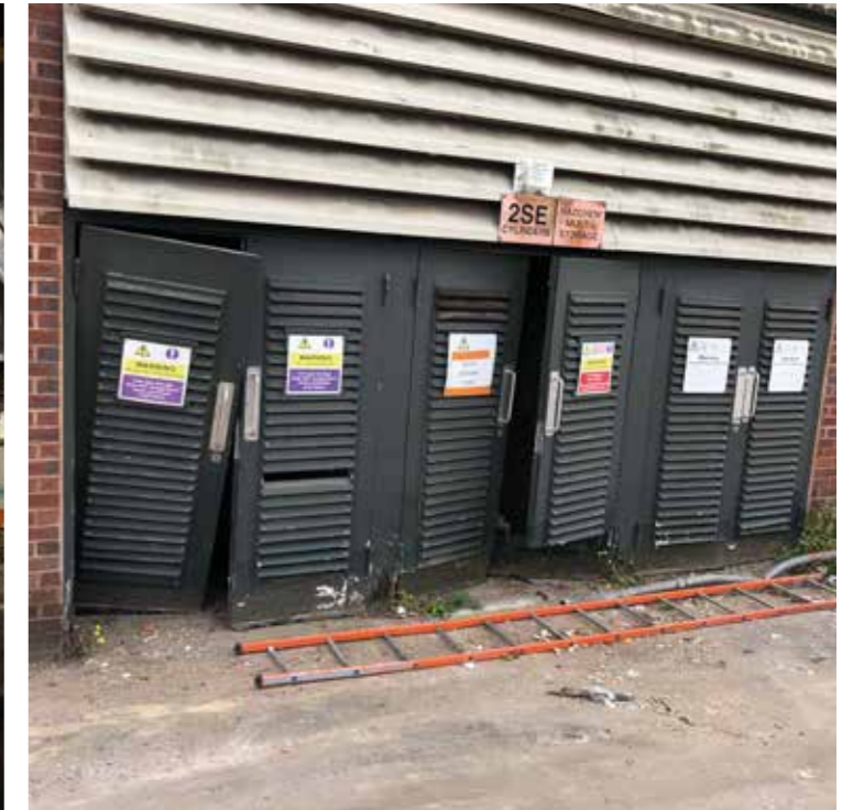
Emptied chemical storage sheds at brewhouse
