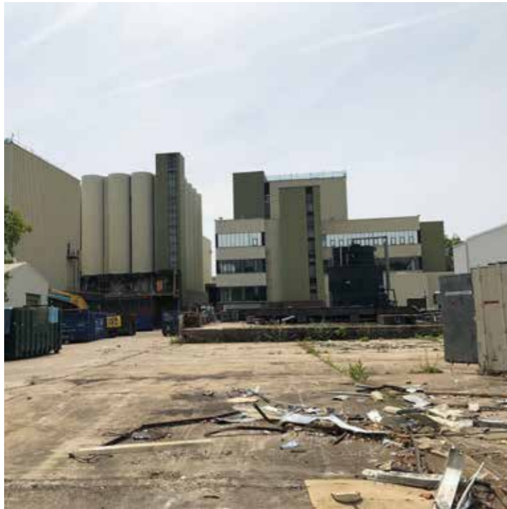
Former base for removed effluent tank
