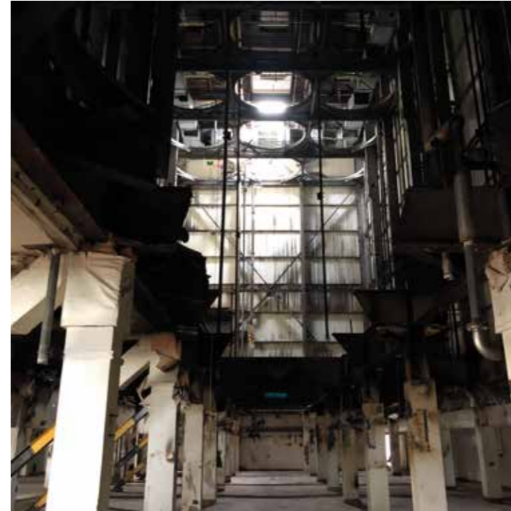
Former tank holders at brewhouse in eastern area
