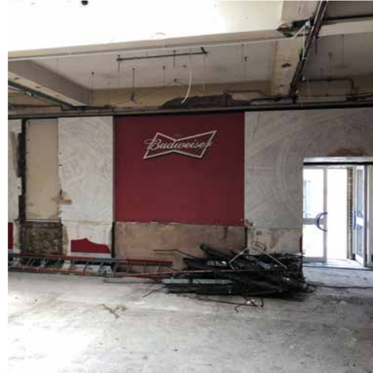
Stripout completed at eastern area canteen building
