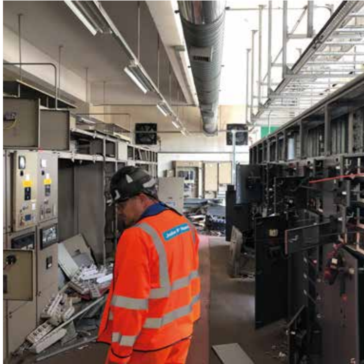
Stripout in progress at energy centre
