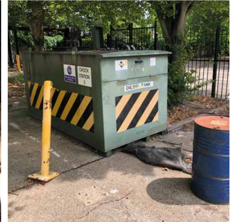
Diesel tank at north of eastern area
