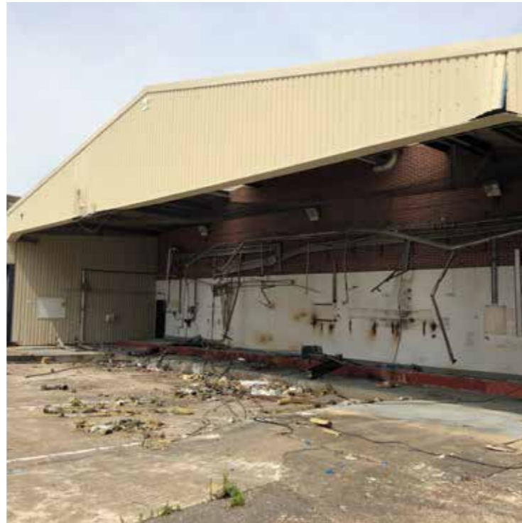
Equipment stripped out of maintenance sheds at western area
