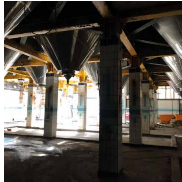
Further tanks in brewhouse awaiting removal
