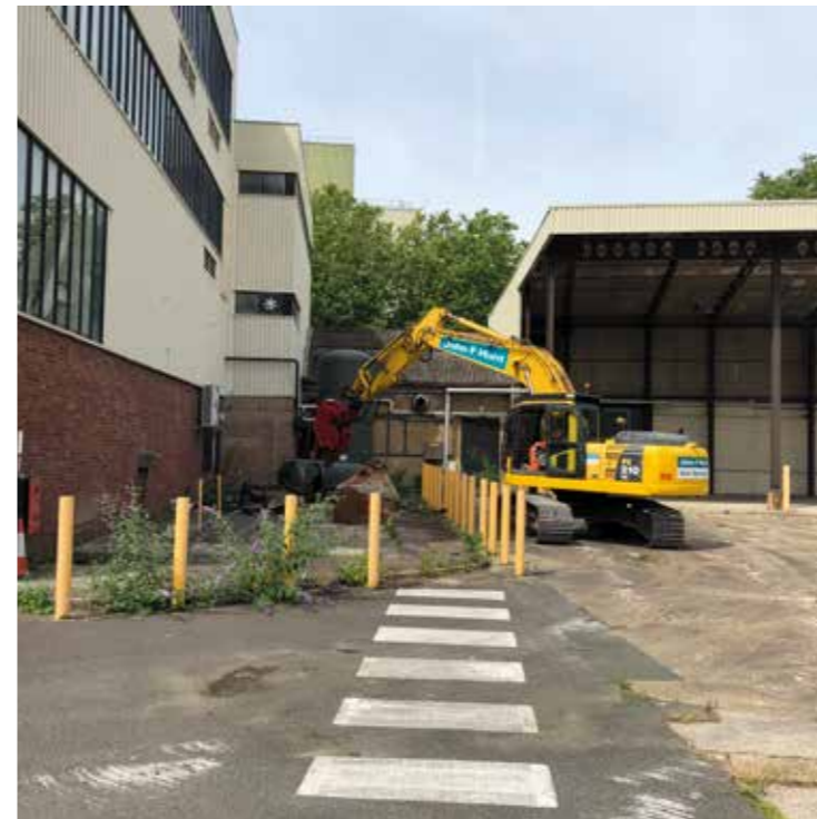
Removal of tanks adjacent to energy centre in progress
