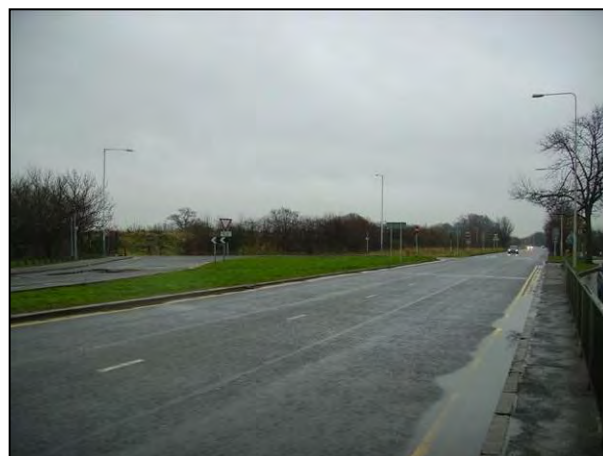
Plate 11: View of Freezeland Way – direction east
