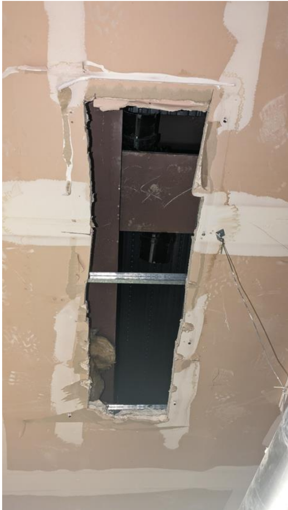
Figure 3 - Steel frame structure seen from ground floor of entertainment building
