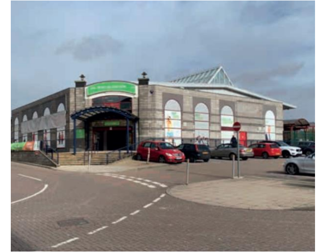
Image 4: Existing leisure centre building
