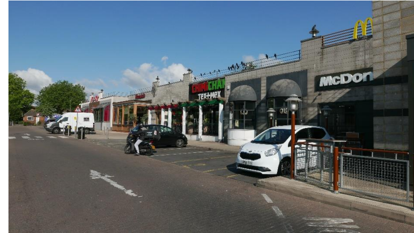
Image 3: Existing restaurant buildings
