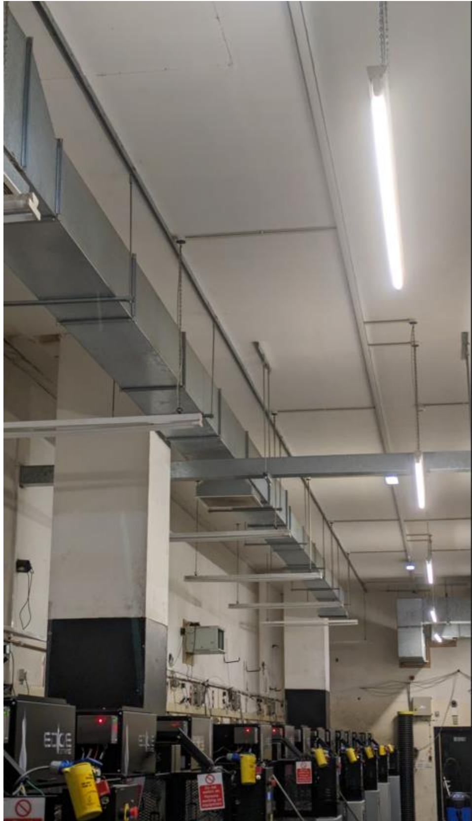
Figure 2 – Steel encased columns from inside of entertainment building
