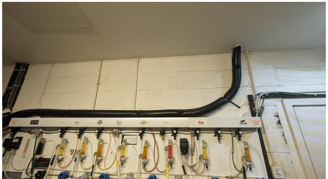
Figure 5 - Blockwork wall viewed internally
