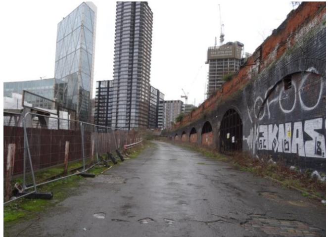
Photograph 5: Area A southern elevation of the tunnels in the south of the site adjacent to railway lines.
