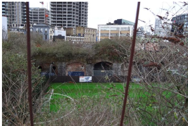
Photograph 12: Tunnels located in Area D (not accessed)
