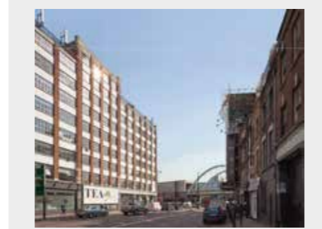
35 | Shoreditch High Street, west side opposite Redchurch Street
