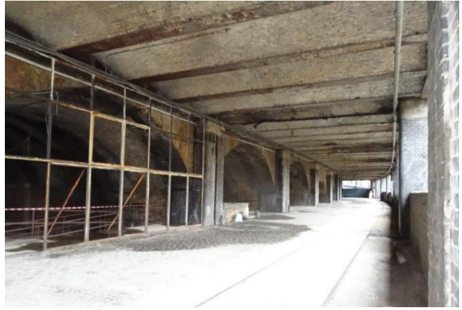
Photograph 7: Eastern section of BPZ2.
