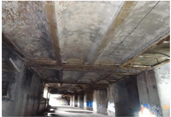
Photograph 1 BPZ1 main tunnel / viaduct with nine tunnels on the right.
