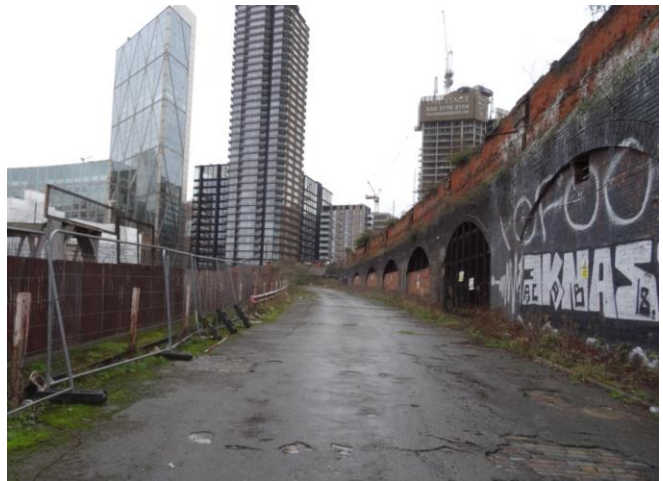
Photograph 5: BPZ1 southern elevation of the tunnels in the south of the site adjacent to railway lines.
