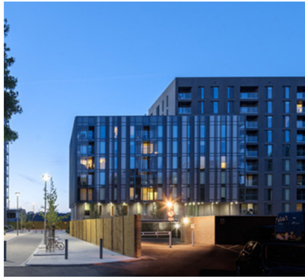
Chambers Wharf, London
