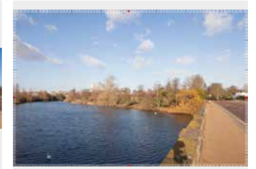
5.1 | Hyde Park / Kensington Gardens: the Serpentine Bridge | Winter
