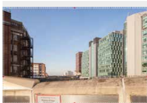
32 | Bishops Bridge Road
