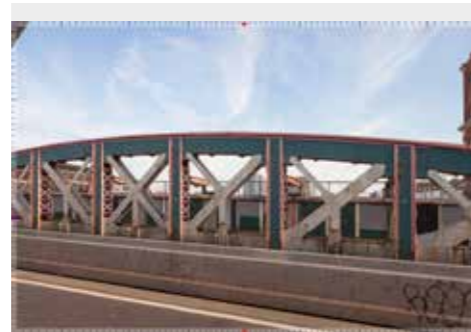
27 | Porchester Road Bridge
