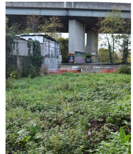
5. York Road (view looking west beneath north circular)
