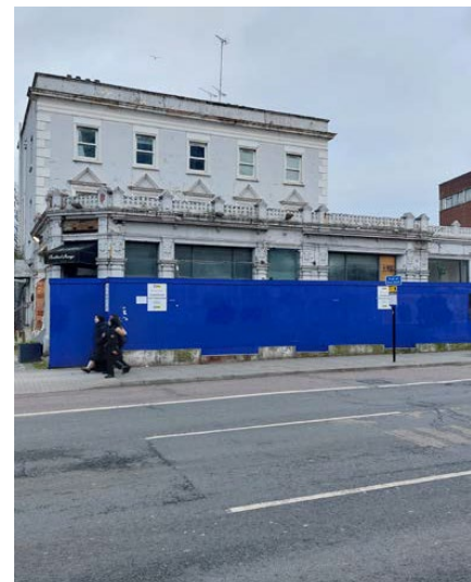
4. Former If Bar Building
