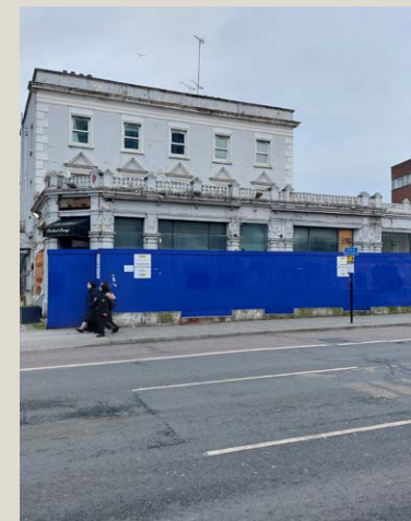
4. Former If Bar Building
