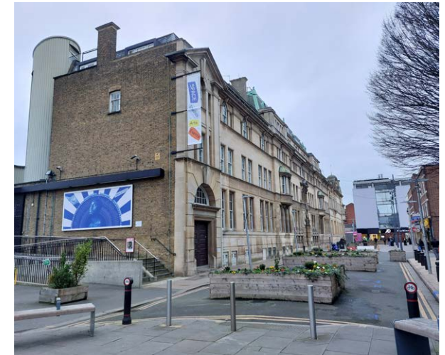
Site 6: Redbridge Town Hall - high retrofit potential
