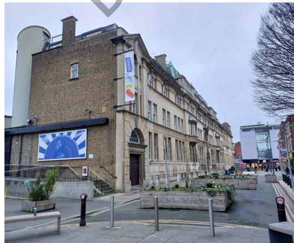
Site 6: Redbridge Town Hall - high retrofit potential
