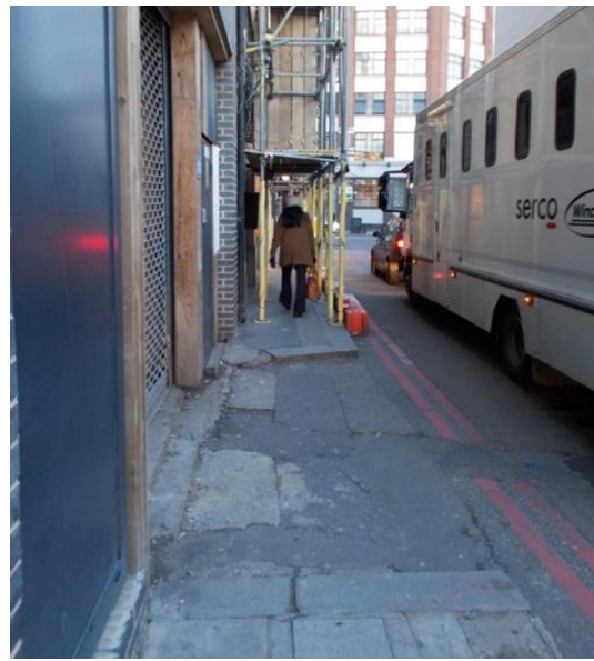
Plate 9 – View of Link L20 (eastwards), trip hazards and narrow effective width caused by presence of temporary scaffolding
