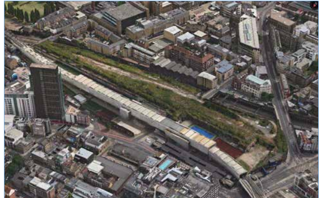
Figure 31 – Existing Site Condition
