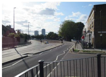
11 Fig.41 Looking west along Abbott Road and the ramp to the vehicle underpass
