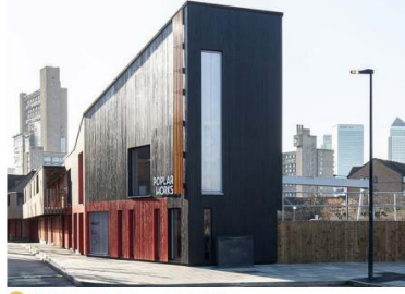
14 Fig.44 Poplar Works development along Naim Street
