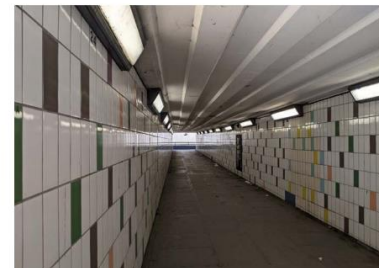
9 Fig.39 Pedestrian underpass under the A12
