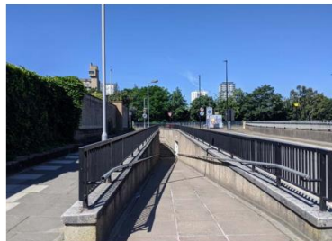
8 Fig.38 Entrance to pedestrian underpass on Abbott Road
