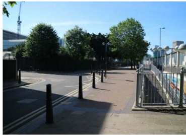
5 Fig.35 Dee Street pedestrian underpass
