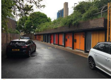
13 Fig.43 Poplar Works development along Naim Street
