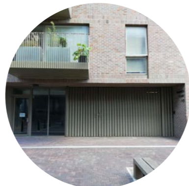
Ancillary spaces are accessible from the street to create activity and have perforated metal frontages
