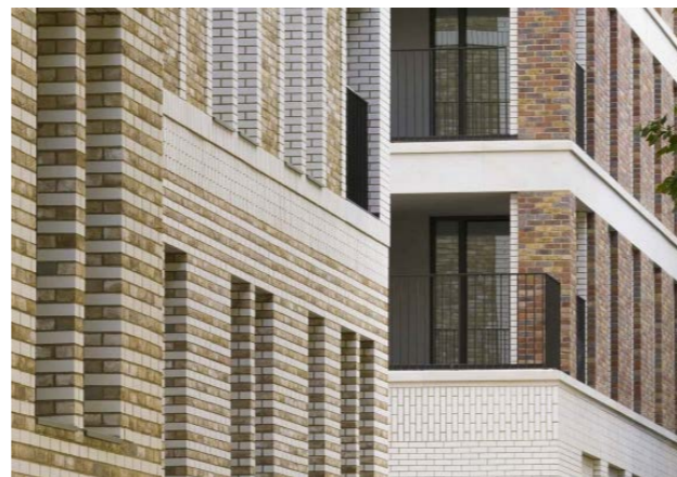
Fig.372 Muted brick tones with concrete banding
