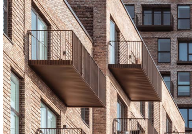
Fig.393 Projecting metal balconies
