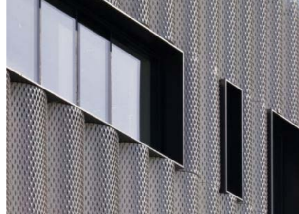
Fig.424 Corrugated-perforated metal cladding
