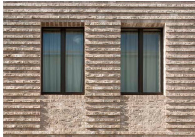
Fig.392 Detail used to expressed oversized window opening
