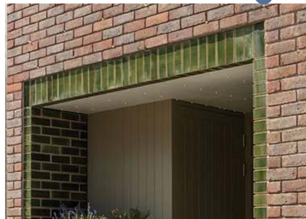
Fig.417 Glazed brick entrances
