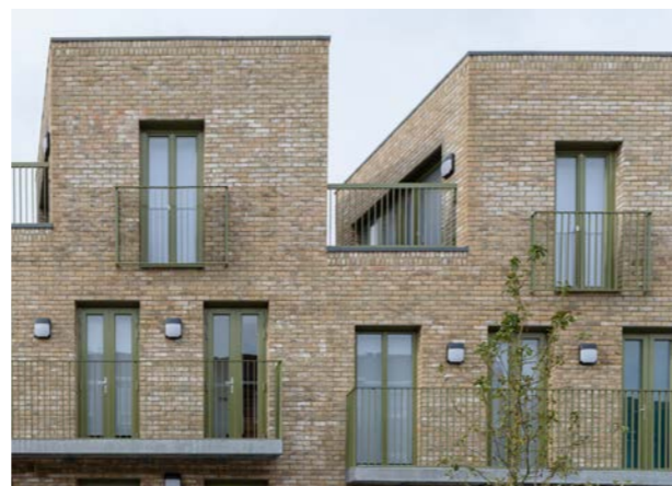
Fig.418 Variation in roof form and use of colour metalwork to match window frame palette
