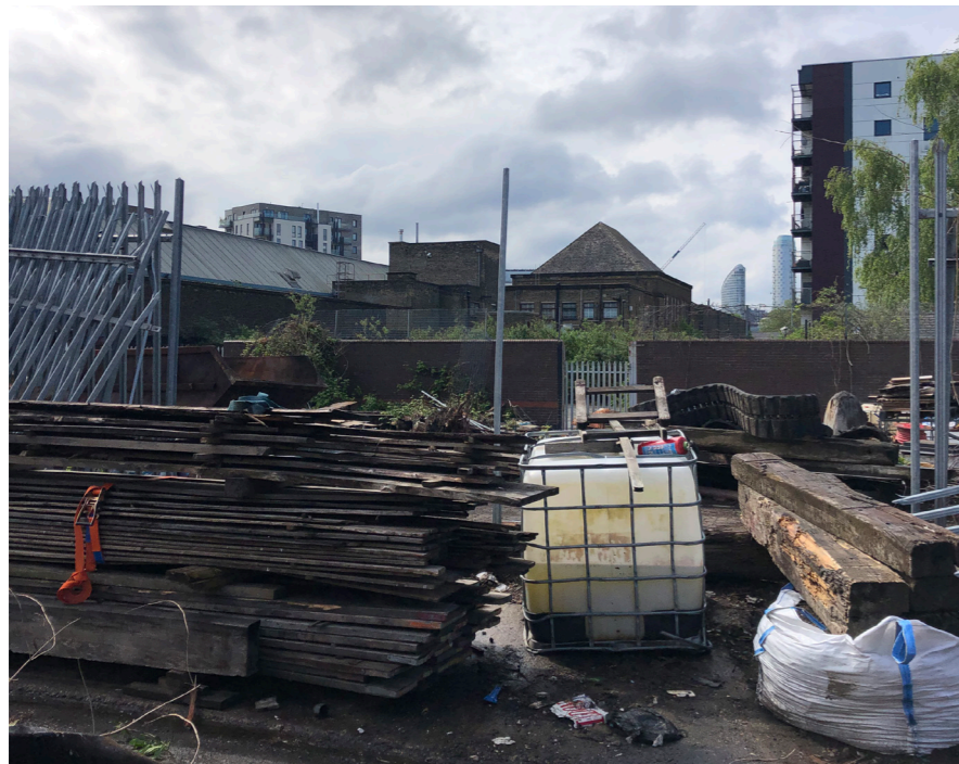
1 View of the existing empty condition looking South from the Eastern end of Plot J
