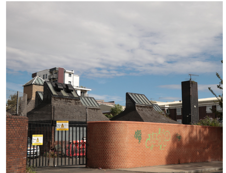
3 Grade II listed Bromley Hall School
