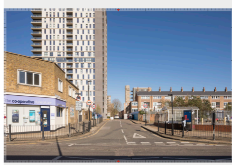
29 | Crisp Street, looking along Willis Street
