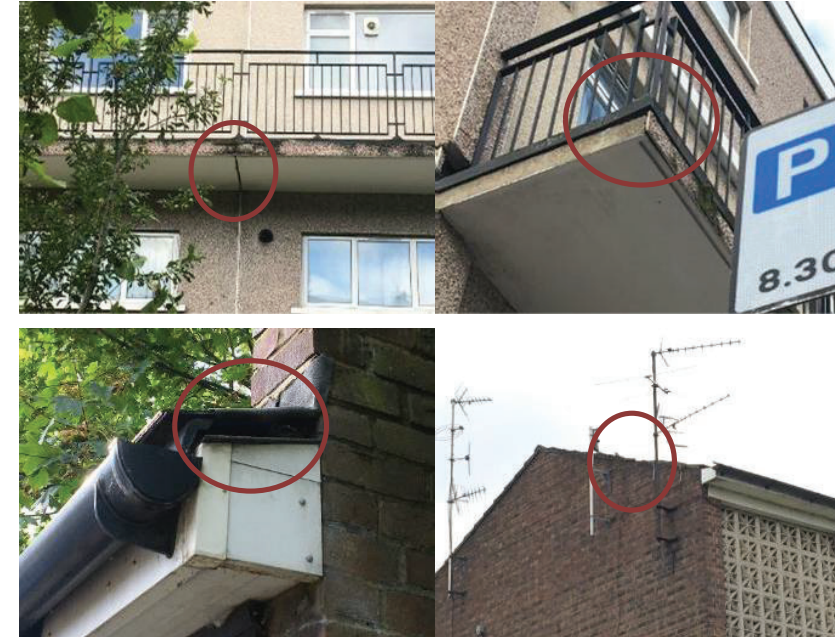
Figure 4.7 Potential roosting features within the built form
