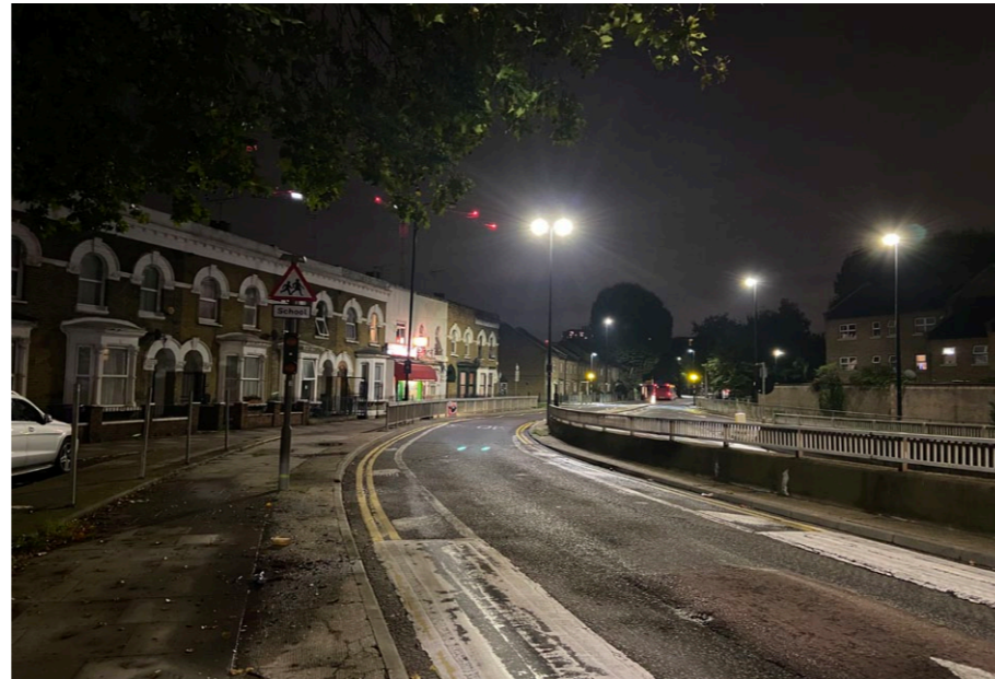
ABBOTT ROAD LOOKING SOUTH
