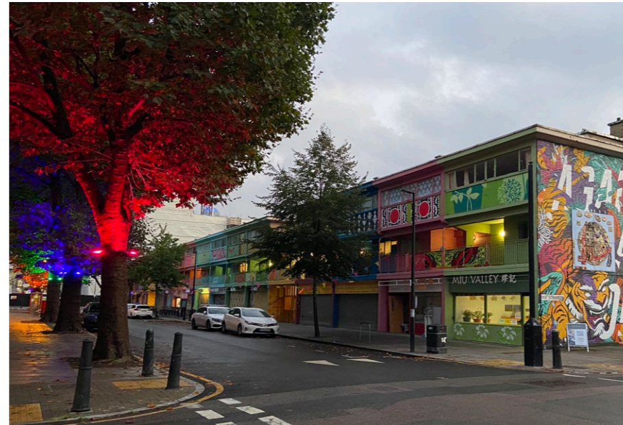
ABERFELDY STREET LOOKING SOUTH
