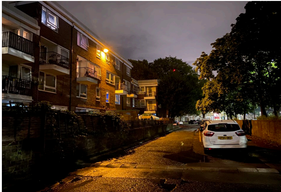
ABBOTT ROAD LOOKING EAST
