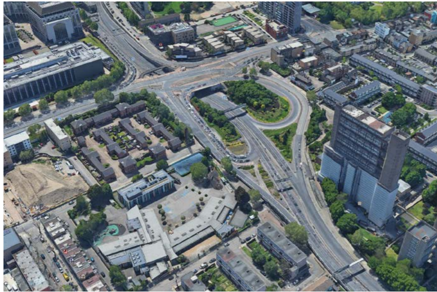
1 Fig.125 Aerial view of the large junction between A12 and A13 towards the Blackwall Tunnel
