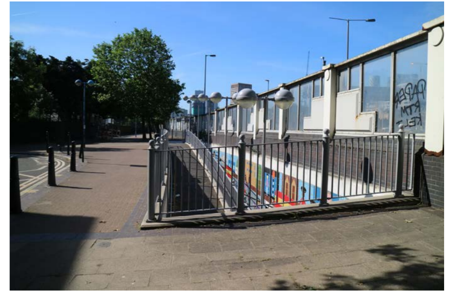
3 Fig.127 The pedestrian underpass at Dee Street
