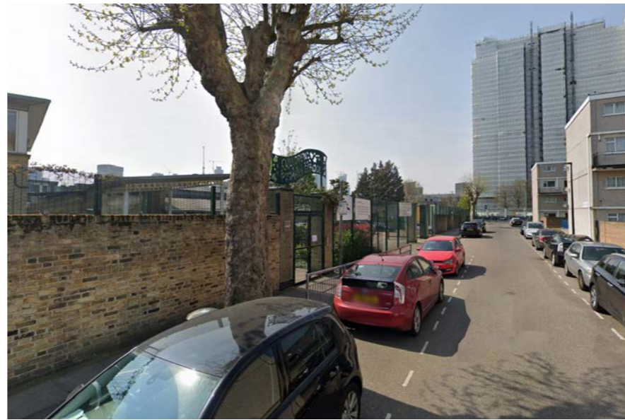
5 Fig.129 Culloden Primary Academy main entrance along Dee Street
