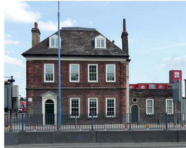
2 Fig.105 Bromley Hall: Grade II* listed building thought to be the oldest brick house in London built in approximately 1485 by Holy Trinity Priory
