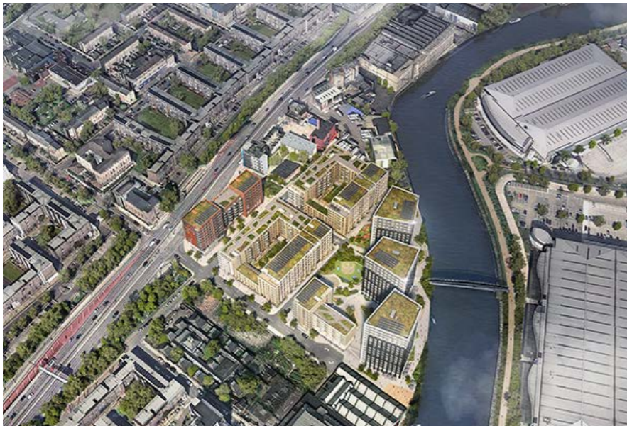
Fig.76 New development adjacent to the River Lea
