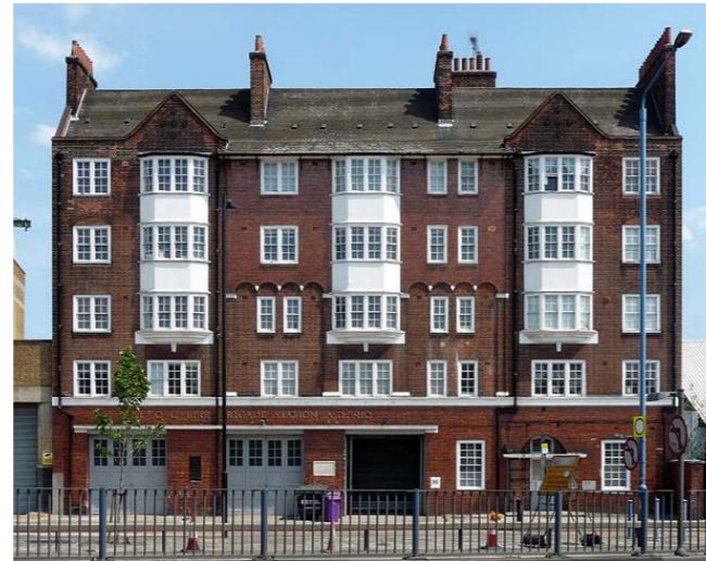
1 Fig.104 Former Fire Station: Grade II listed fire station built in 1910 and designed by London County Architects
