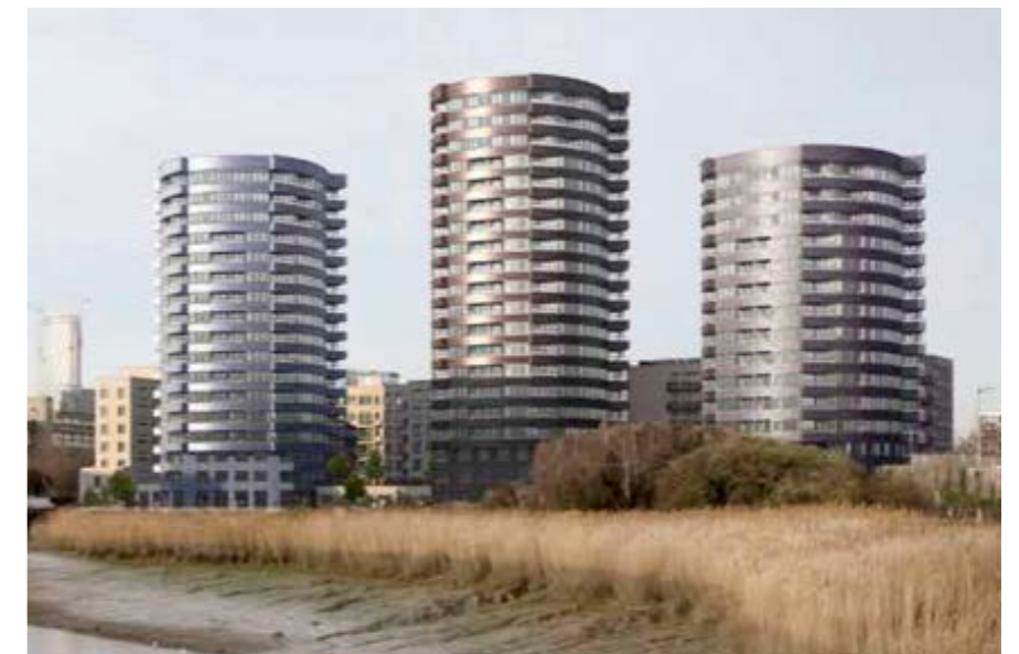
5 Fig.88 East Riverside / Former Poplar Bus Depot: 15, 17 and 20 storeys/ up to 72.2m AOD
