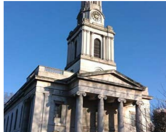
12 Fig.115 All Saints Church with St Frideswide: Grade II listed church built in 1817 and designed by J Hollis
