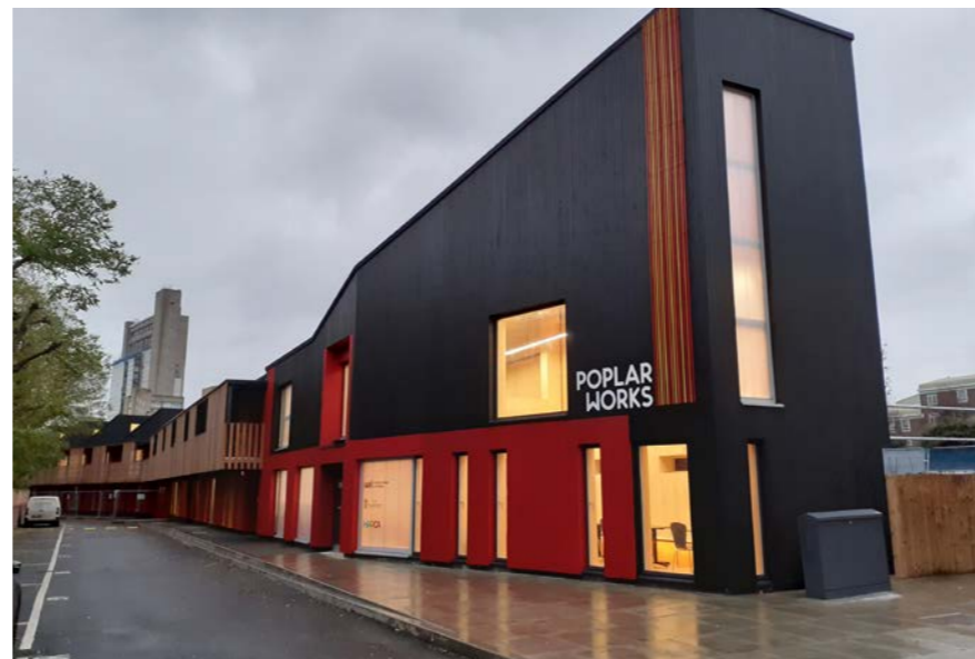
5 Fig.94 Recently completed Poplar Works offering small affordable workspaces to creatives
