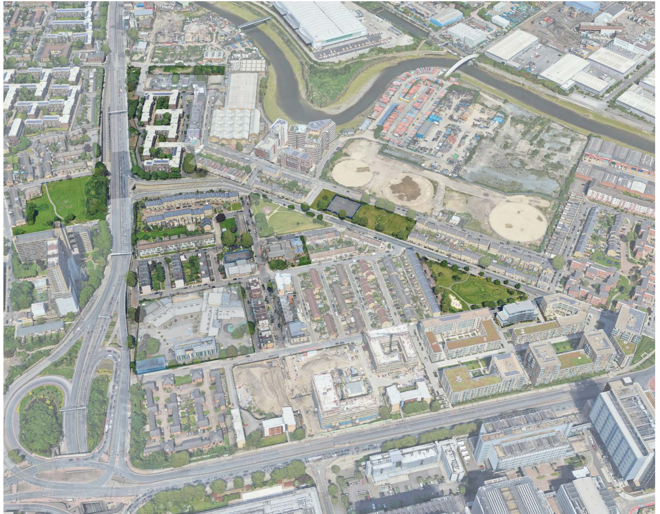
Fig.82 Aerial view of the site early 2019
