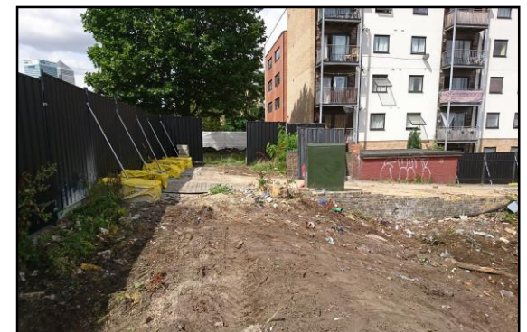
Surface scraped off towards substation area
