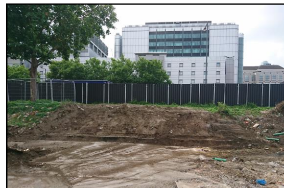
On completion of 14t work
