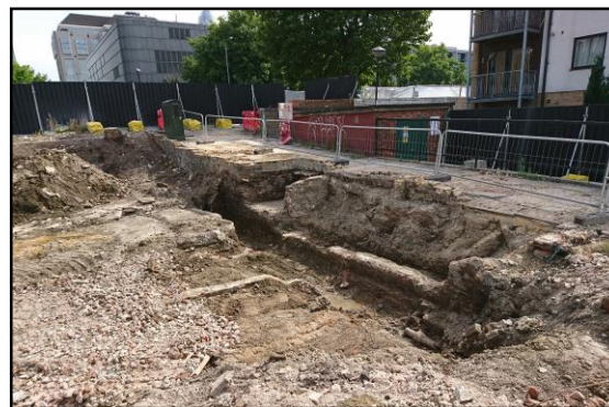
General area showing buried walls and footings
