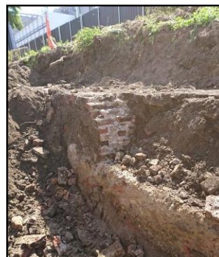
Footings encountered during excavation
