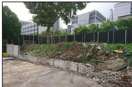
Area before excavation
