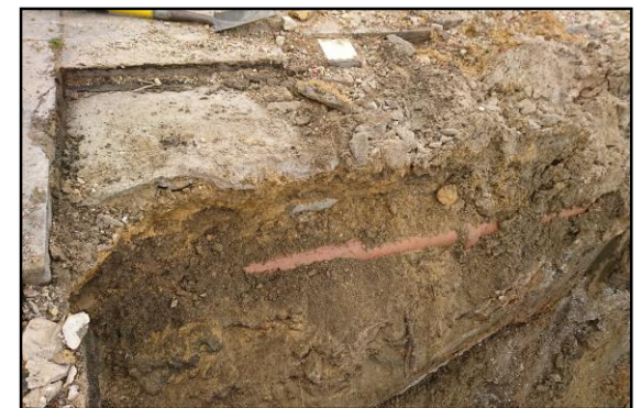
Chasing out around services by hand
