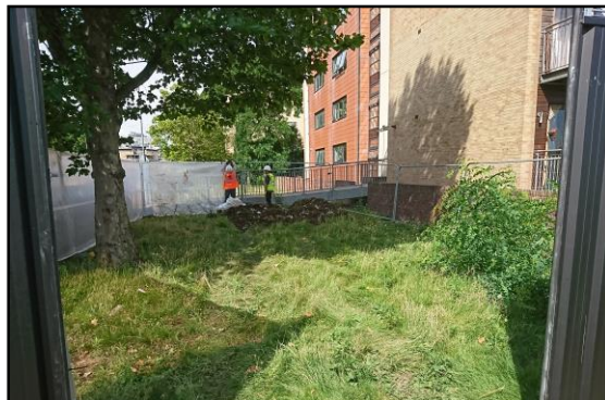
Temporary fence being installed
