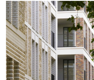
Fig.75 Horizontal concrete banding within brick façade
