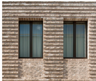
Fig.67 Recessed and banded brickwork detail
