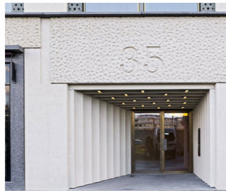
Fig.85 Clearly defined residential entrance
