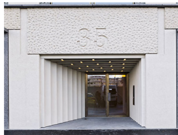
Fig.189 Pale concrete base with sculptural residential entrance
