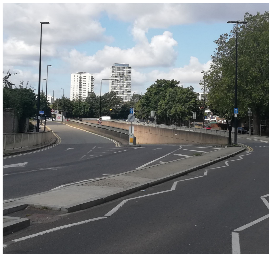
11 Fig.19 Vehicular underpass along Abbott Road crossing the A12. This creates a barrier between Aberfeldy Estate to the south and Nairn Street Estate to the north.
