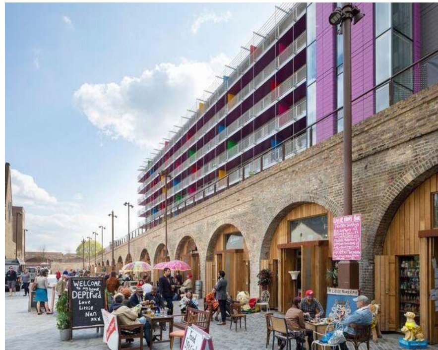
Fig.649 Deptford Arches, Lewisham
