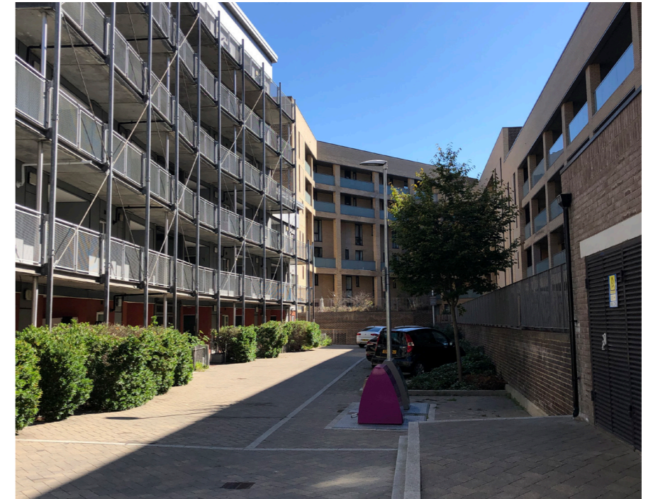
3 View of the existing carpark to the rear of Blairgowrie Court and sub-station / sulo
