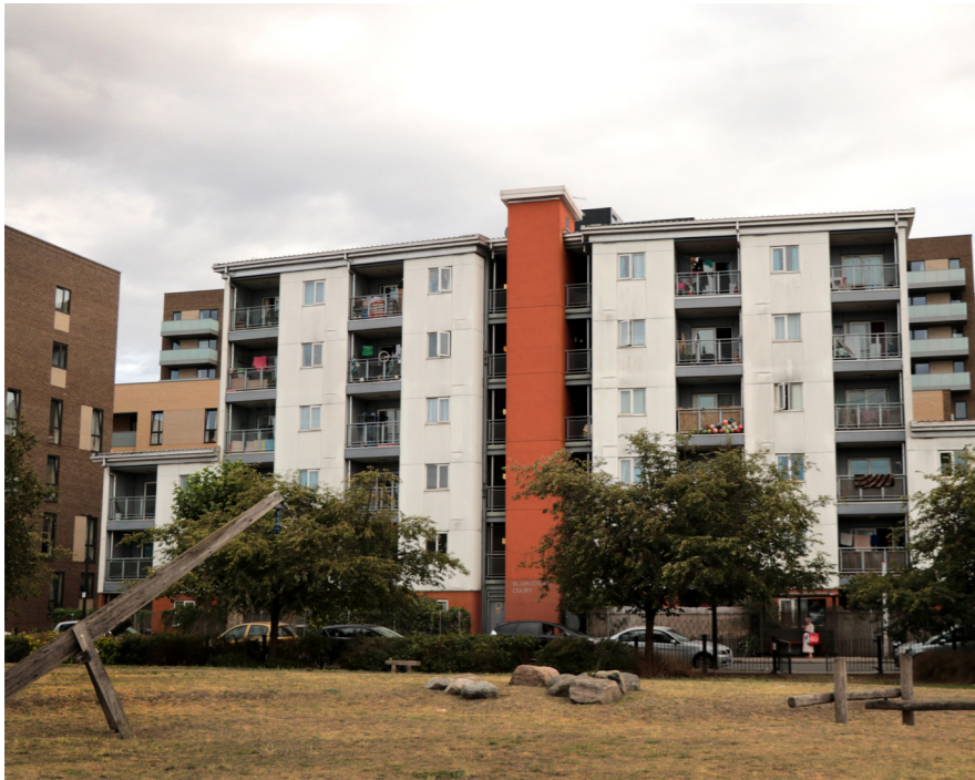
1 View of the Existing Blairgowrie Court to be demolished
