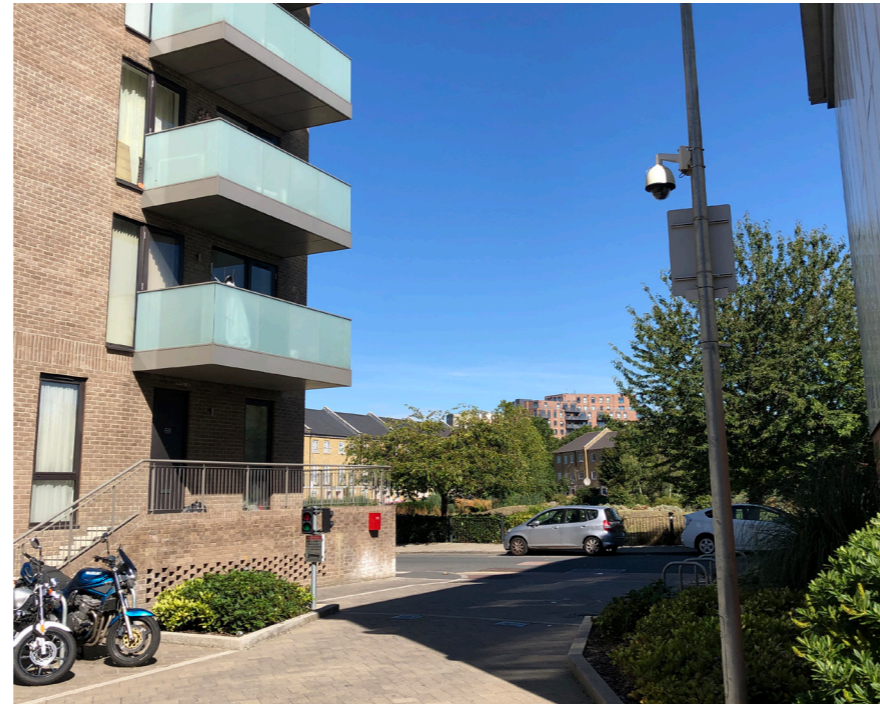
2 View looking North up Blairgowrie Court towards Braithwaite Park
