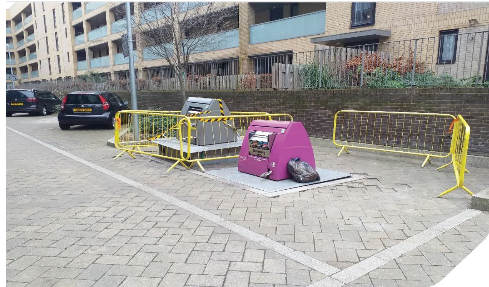
Photo 05: Blairgowrie Park underground waste storage system
