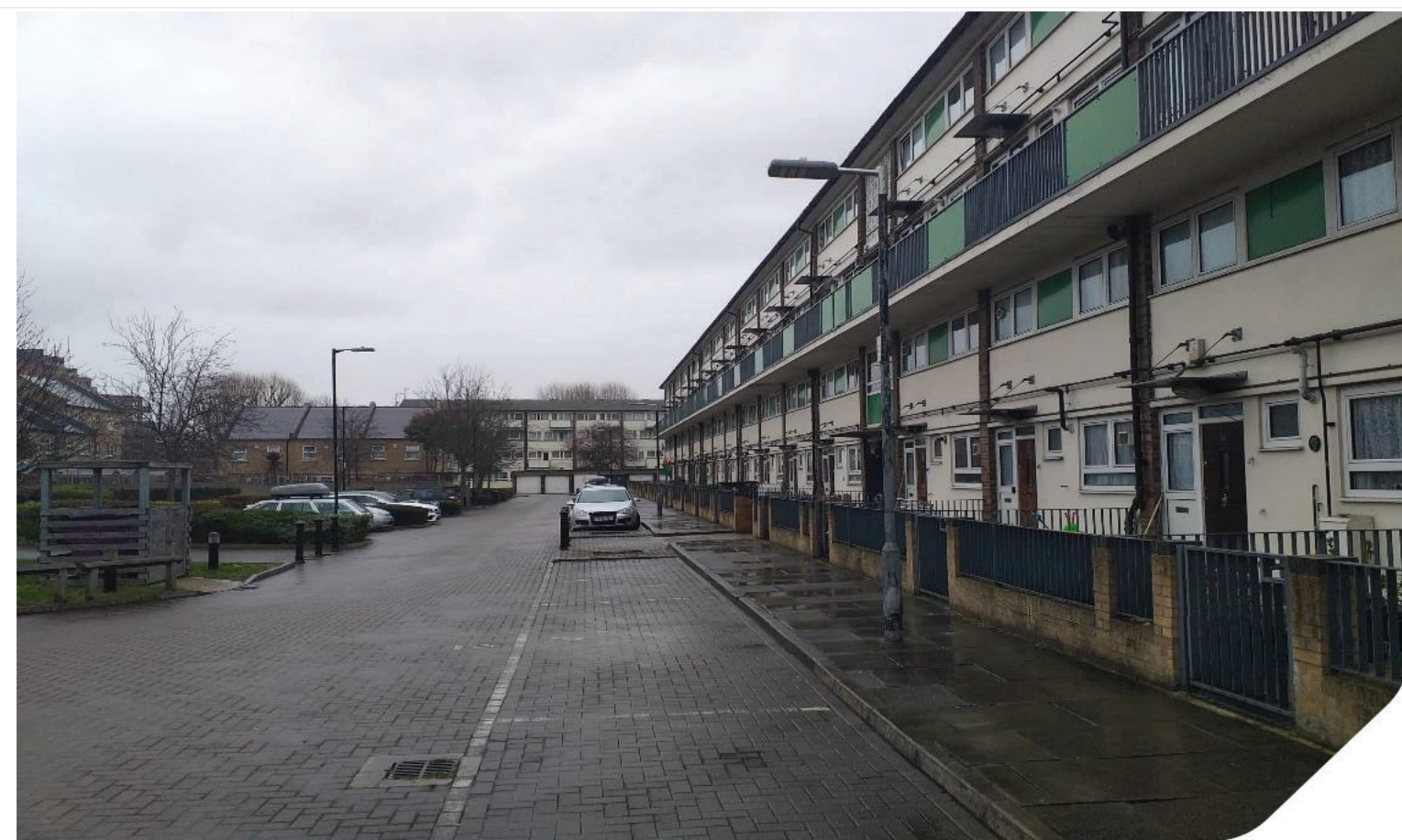
Photo 14: Flats off Findhorn Street
