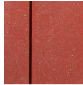
Etched concrete (colour: Terracotta)
