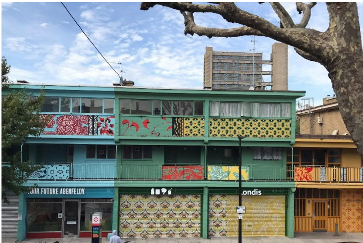
Figure 3-5 Building Exterior – Frontage
