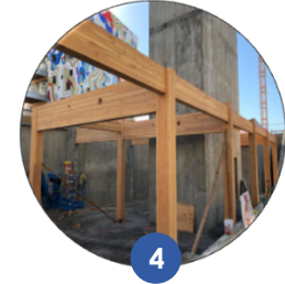
CONCRETE WITH TIMBER INCLUDED With CLT timber deck with Glulam beams for alternate floor levels.
