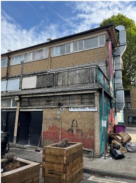
Figure 3-6 Building Exterior - Rear
