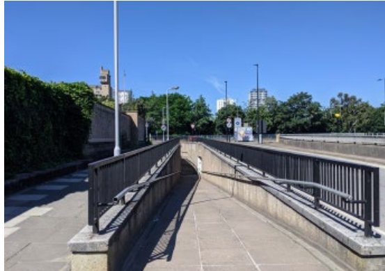
Entrance to pedestrian underpass along Abbott Road
