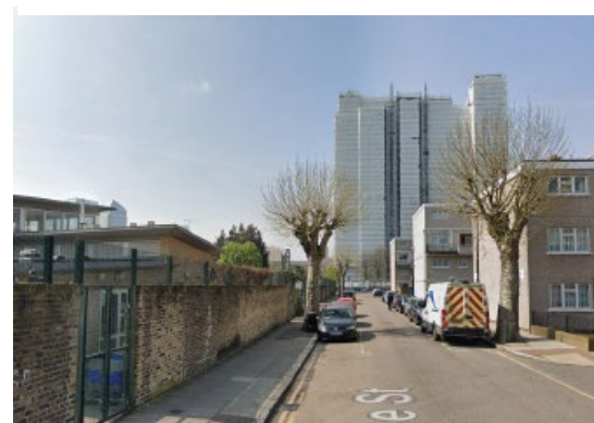
View along Dee Street to Balfron Tower
