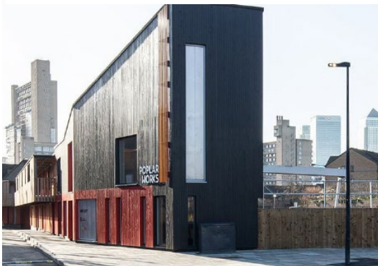
Poplar Works development along Nairn Street
