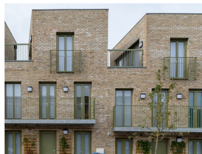
Fig.253 Variation in roof form and use of coloured metalwork
