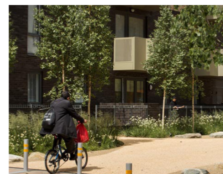
Fig.245 Generous paths and tree planting through Ocean Estate, Stepney Aberfeldy Village Masterplan Design Code Revision D
