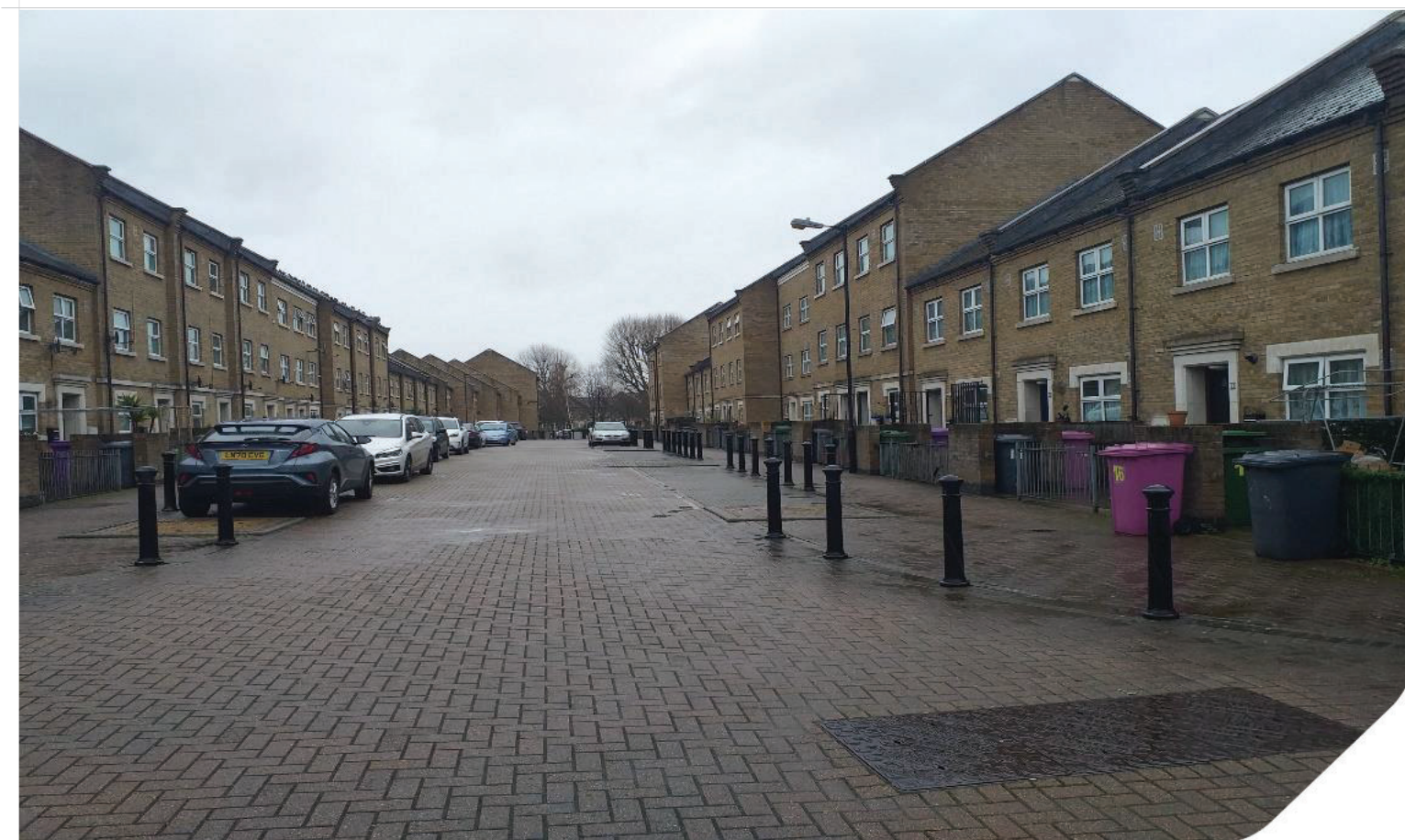
Photo 15: Residential Properties along Balmore Close
