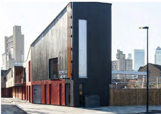
Poplar Works development along Nairn Street
