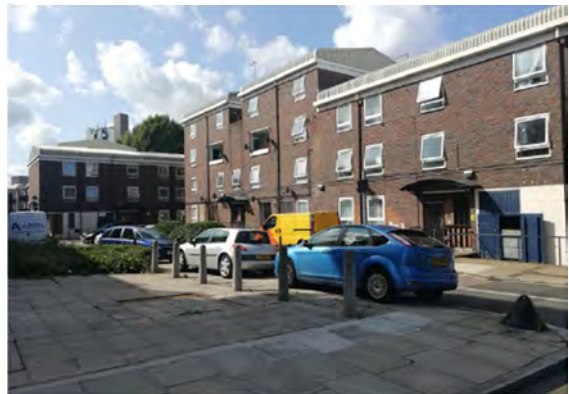
Looking south along Nairn Street
