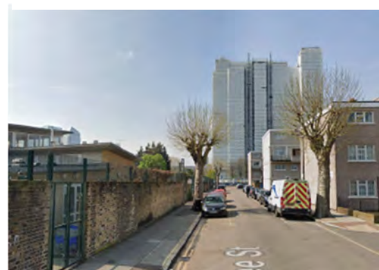
View along Dee Street to Balfron Tower
