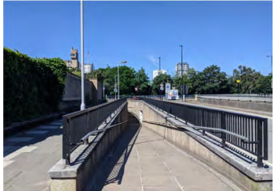
Entrance to pedestrian underpass along Abbott Road
