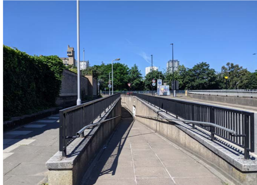
8 Fig.38 Entrance to pedestrian underpass on Abbott Road
