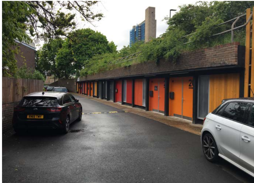
13 Fig.43 Poplar Works development along Nairn Street
