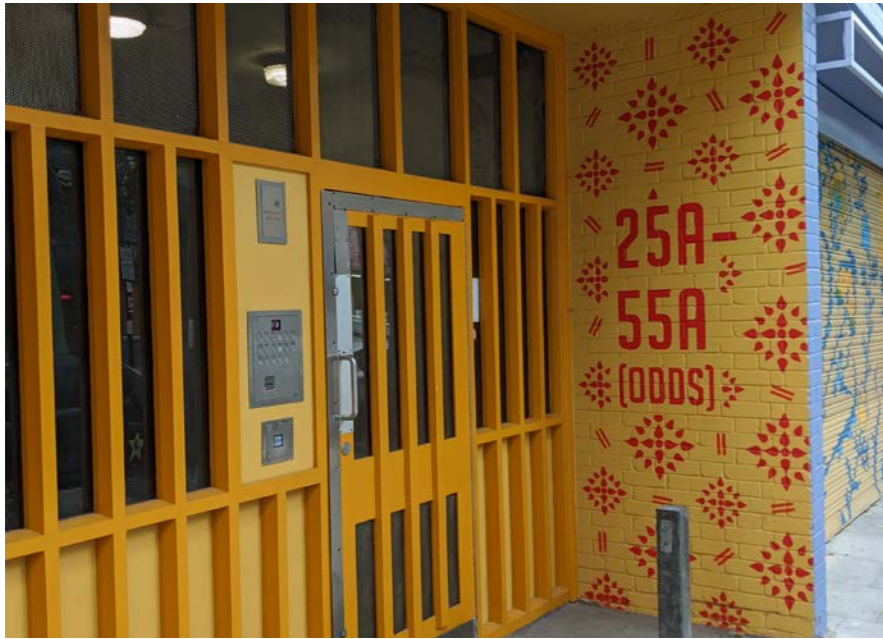
Fig.59 Improvements to signage and entrances and wayfinding
