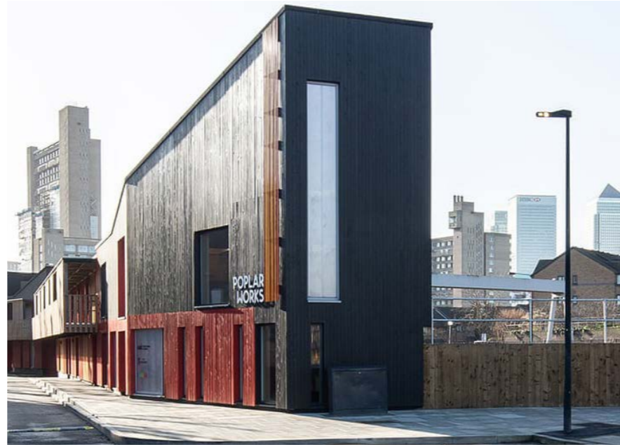
14 Fig.44 Poplar Works development along Nairn Street
