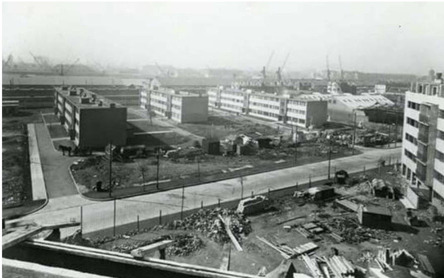
Fig.25 Aerial view from Abbott Road towards the new residential estate
