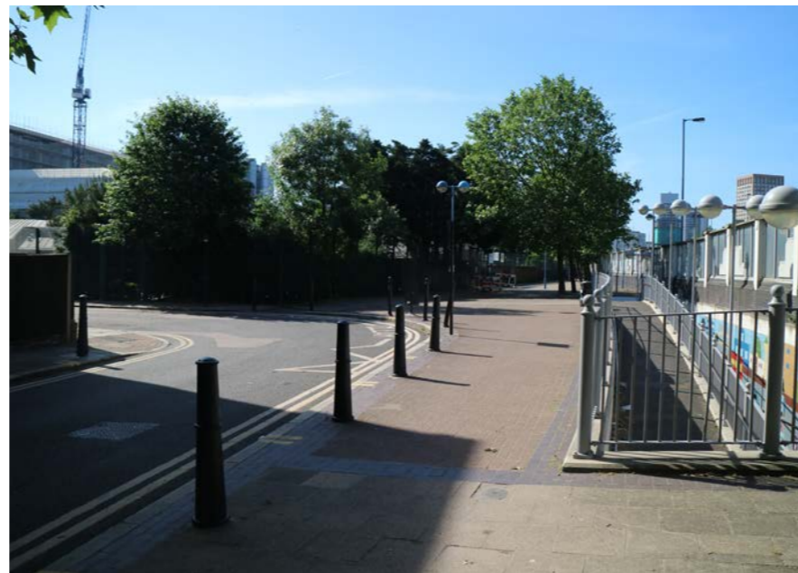
5 Fig.35 Dee Street pedestrian underpass
