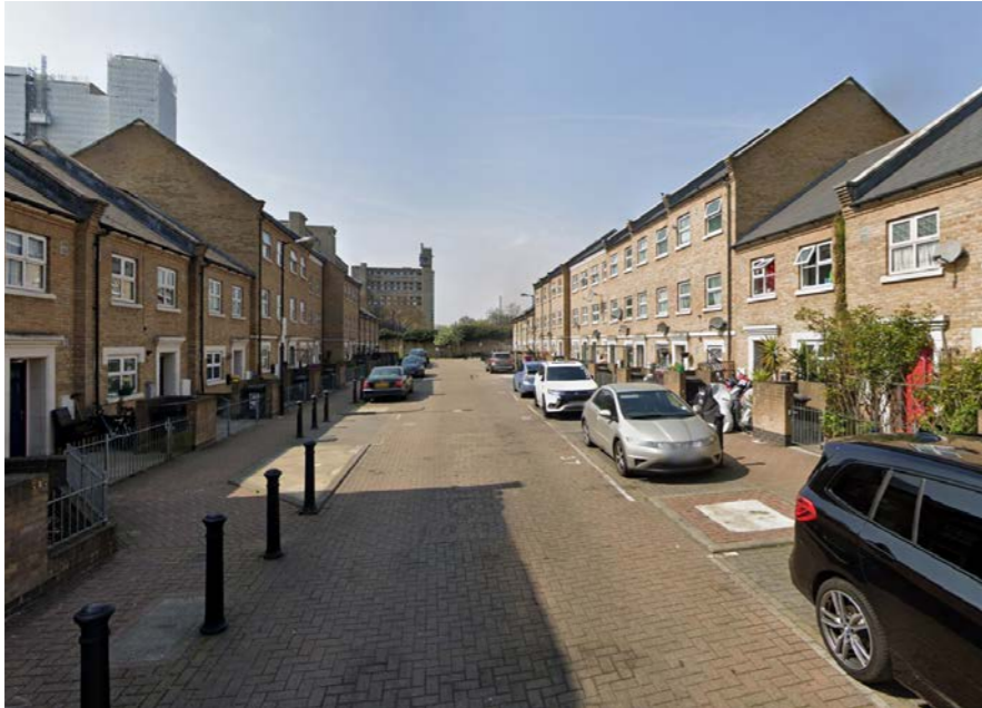
7 Fig.37 View looking west along Balmore Close
