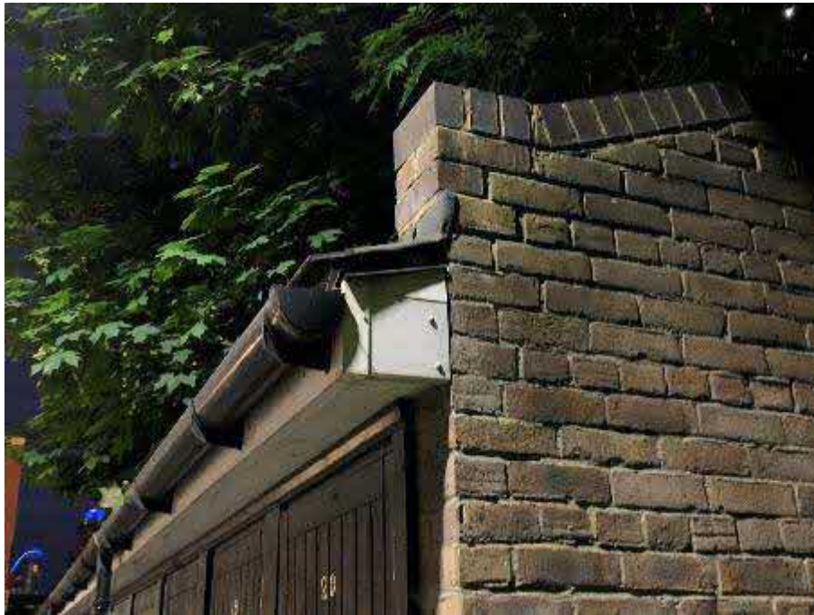
Figure 4.2 Lighting of potential roosting features on site
