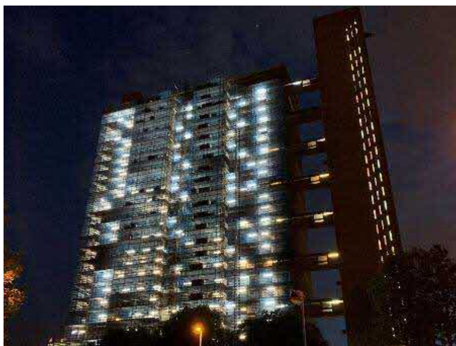
Figure 4.2 External lighting in the area which is likely prohibitive to bats
