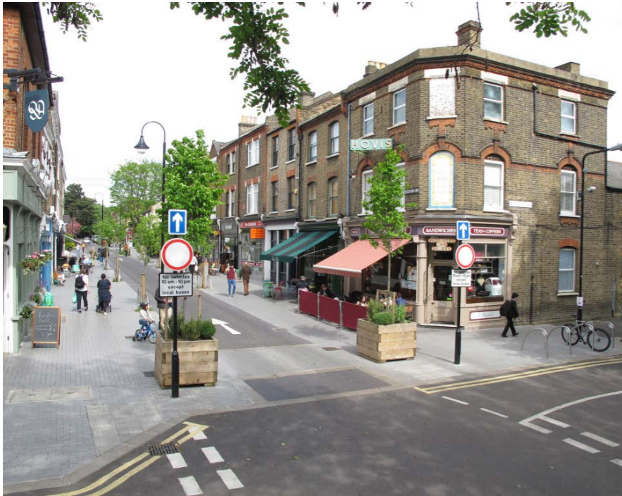
Fig.485 Generous pavements and motorist de-prioritisation, Orford Road Walthamstow
