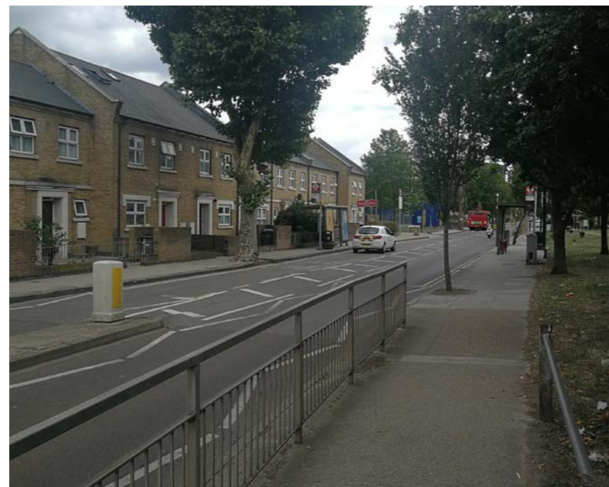
Fig.482 Central reservation in middle of Abbott Road
