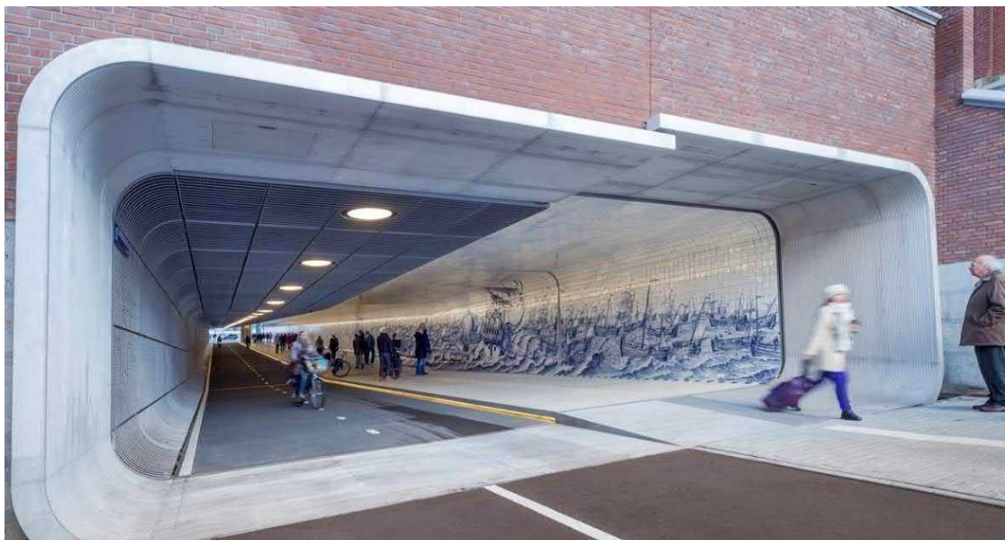
Figure 3-19: Amsterdam Central Station Pedestrian-Cycle Tunnel
