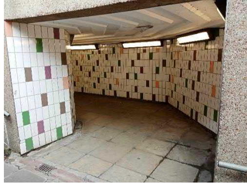
Photo 4: Abbott Road Subway Entrance
