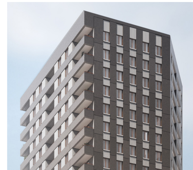
Fig.326 Top of B3 showing contrast between vertical and horizontal façade expression (Illustrative proposal)
