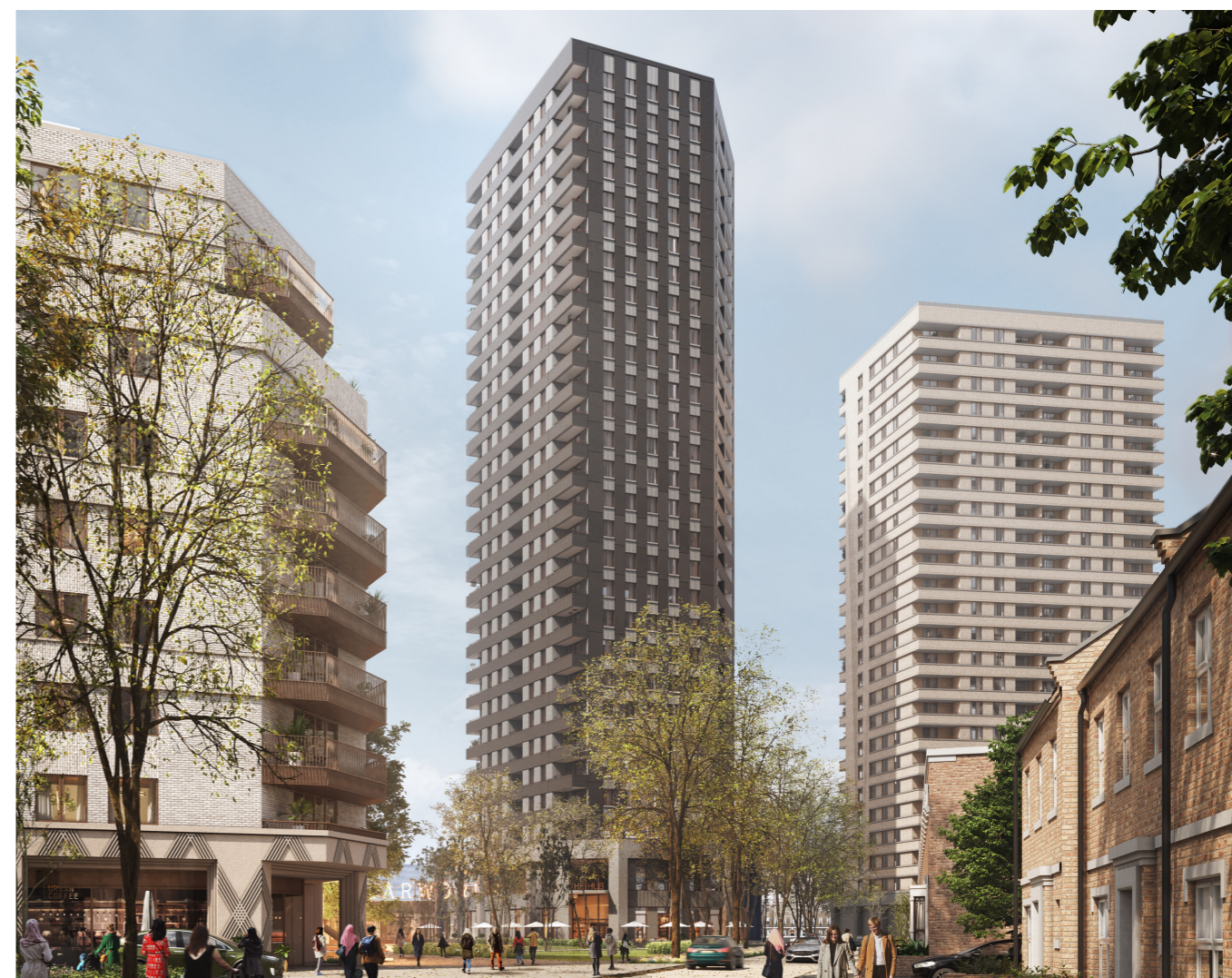
Fig.327 Illustrative view of Building B3 viewed from Abbott Road
