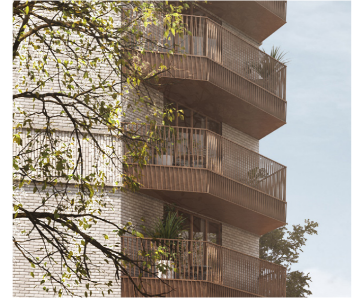
Fig.351 Illustrative view of chamfered corner at upper levels with metal balconies
