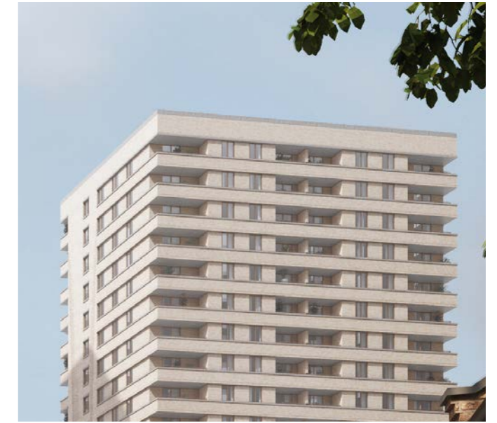
Fig.367 Top of Building B2
