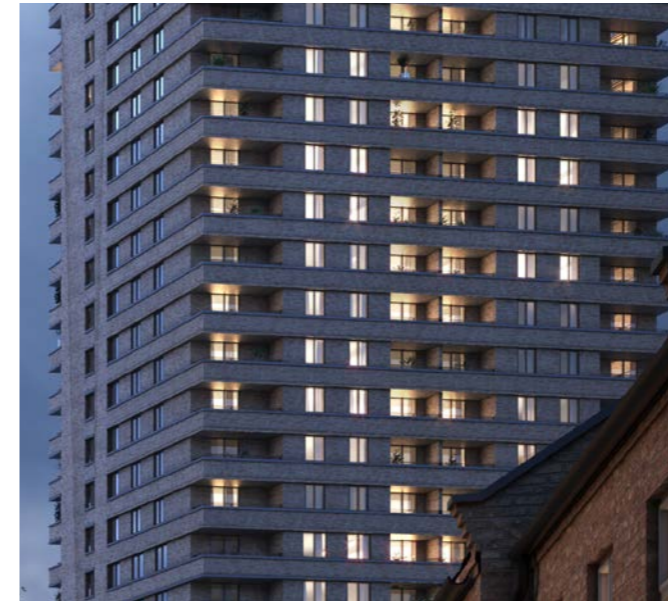
Fig.366 Recessed balconies and concrete banding to Building B2
