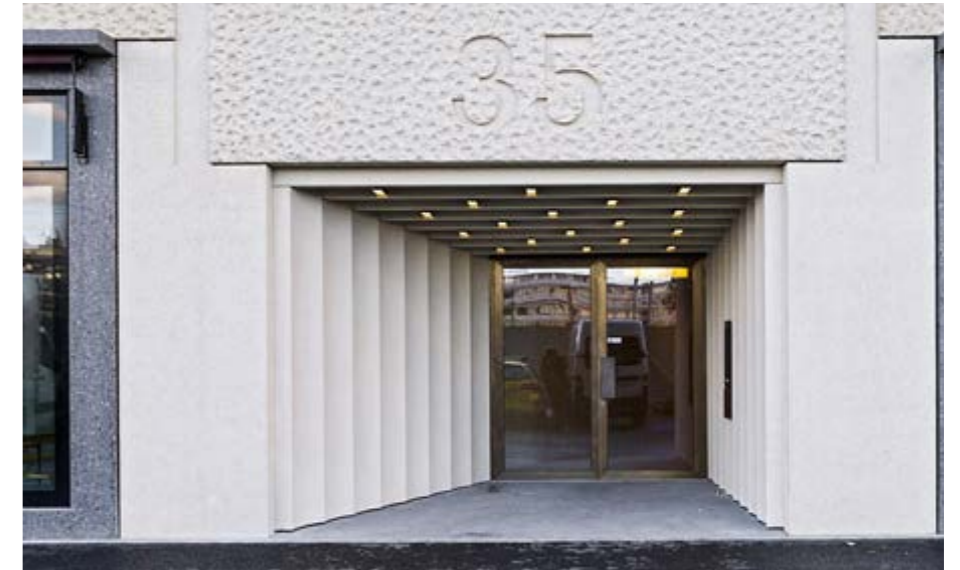
Fig.350 Generous single storey entrances marked with splayed recessed detail, signage and lighting
