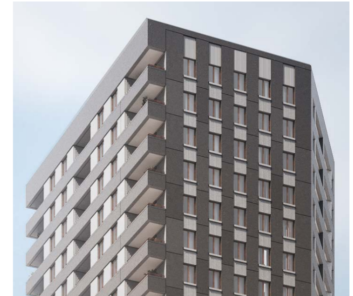
Fig.356 Top of B3 tower showing contrast between vertical and horizontal facade expression
