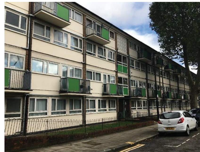
Figure 4.4 Residential flats in the main body of the site
