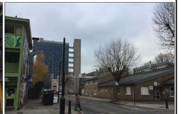
Plate 2. South-west of the site, looking north-west from Blair Street.
