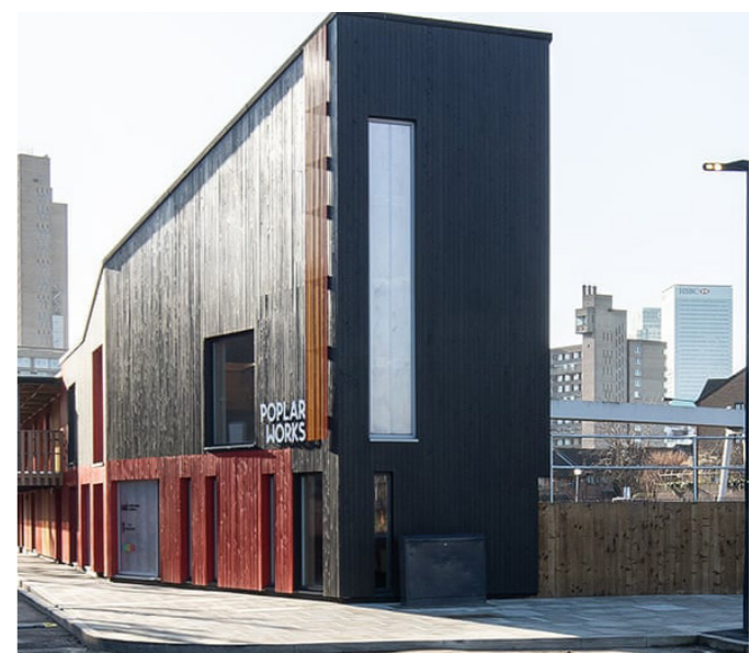
Fig.206 Existing Poplar Works building with dark cladding and playful roof form
