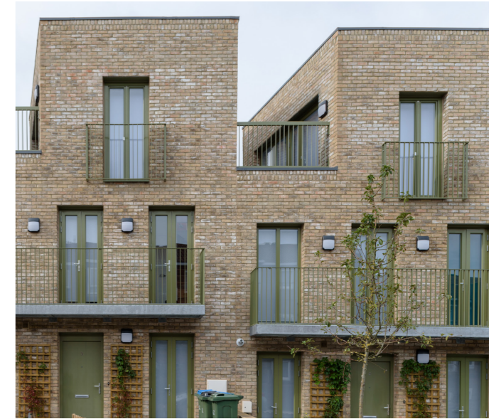
Fig.238 Projecting balconies and coloured metalwork to match window frames
