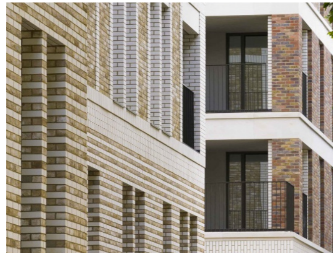
Fig.330 Muted brick tones with horizontal banding
